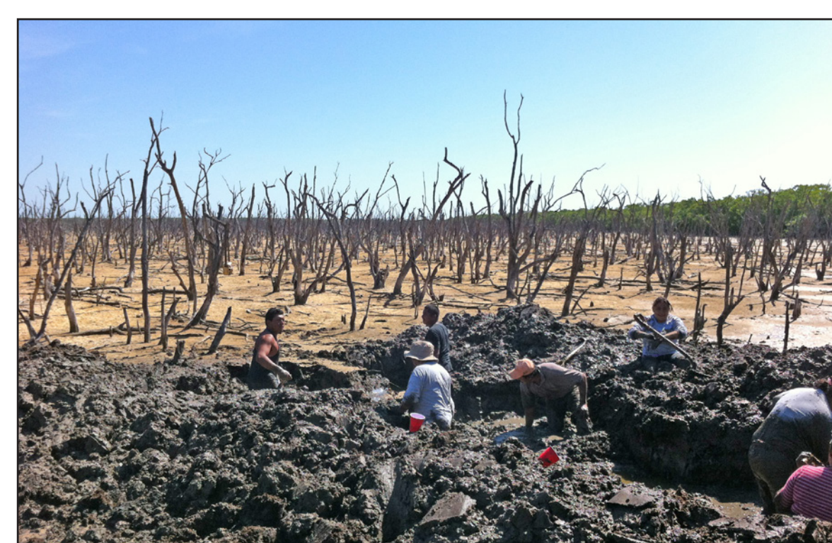
12 project workers hand digging canals to bring water back to area
